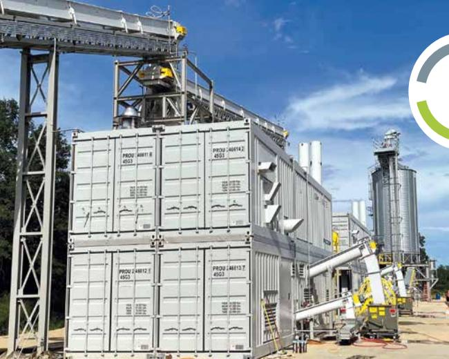
**PelletBOX** is a containerized pellet plant with a capacity of 5 tons per hour of both domestic and industrial pellets.
